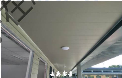
Real Picture of Corridor
