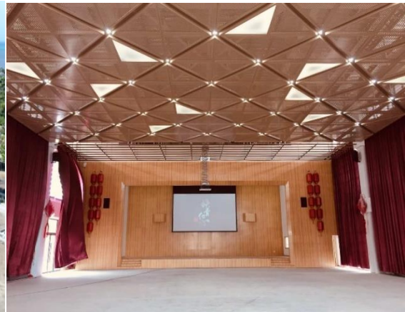
室内安装 Interior Finishing
