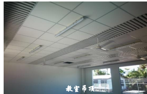
Real Picture of Classroom Ceiling
