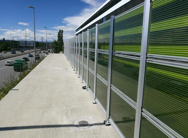
ELECTRIC POWER PRODUCING GREEN NOISE BARRIER INSTALLED AT THE MOTORWAY BETWEEN BERN AND ZURICH
