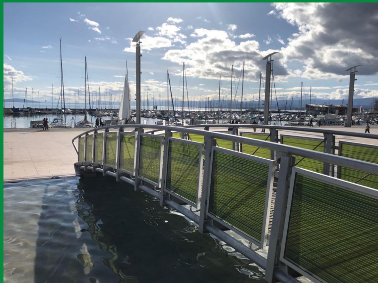
Bridge at lake Geneva in Lausanne
