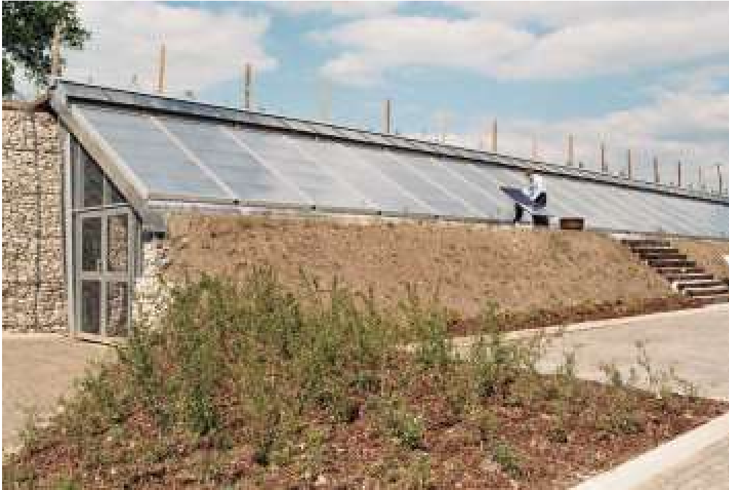
Fig. 2.1. PVT façade at RES UK in Kings Langley (UK). Photograph © Henk Kaan.
